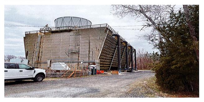
Mr. Irving described the cooling tower. Build in 1972. Size is 48 feet high to deck and another 18 feet for fan stack and is 128 feet in length, 75 feet wide.
