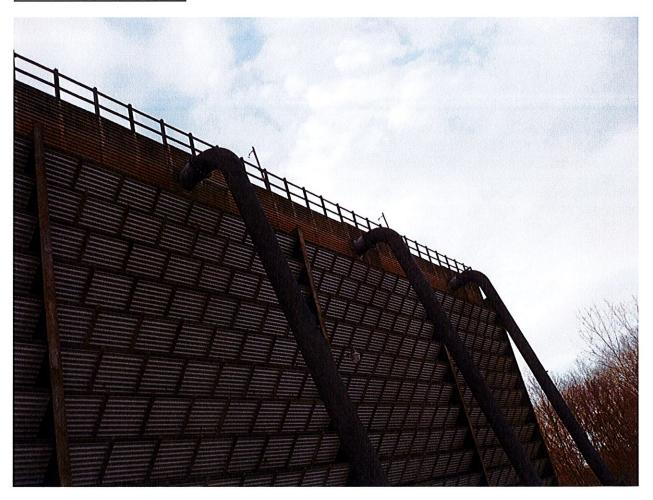
Cooling tower contains 4 cells and 4 fans. Water comes in over the top. Air in or out from the side.
